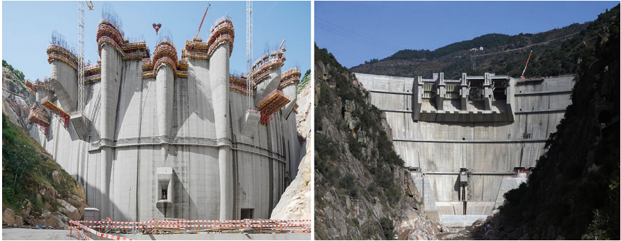
Fig. 2. Upstream view (under construction) and downstream view of Foz Tua dam.
